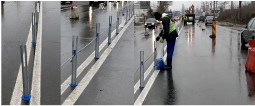
Figure 9. Sector on DN 2 with the cable parapet pilot project.
