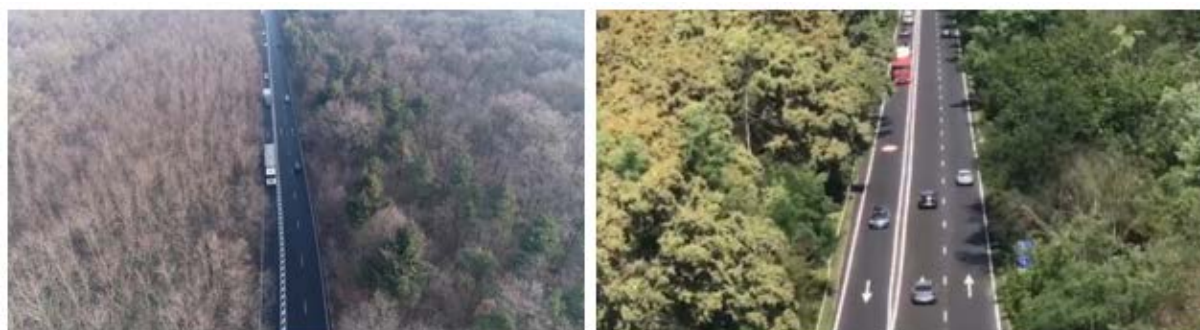
Figure 8. Sector on DN 2 in 2+1 traffic system.
