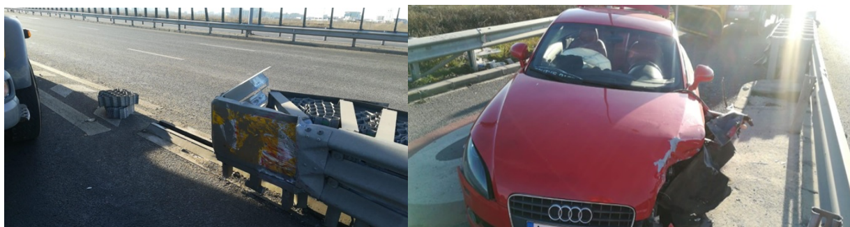
Figure 7. Degraded impact attenuator.
