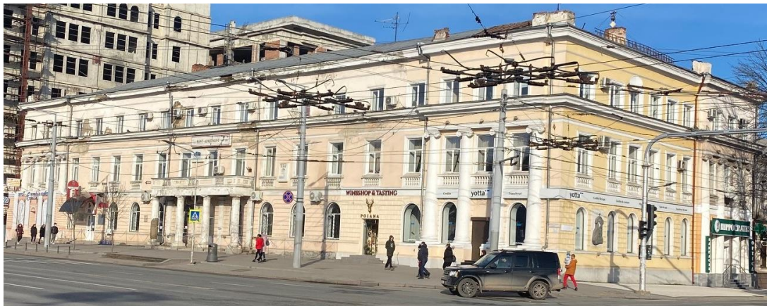
Figure 5. Facade of the historical monument on 148 Stefan cel Mare Boulevard, Chisinau, Republic of Moldova, 2021.
