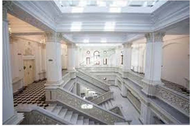
Figure 2. Stairs of the headquarters after the reconstruction of the National Museum of Plastic Arts of Moldova.
