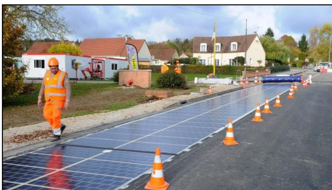
Figure 3. Wattway panels pavement.
